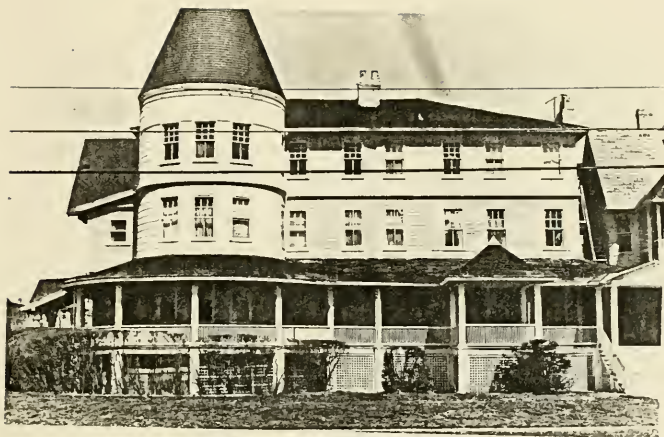
Plate 15: Cottage #1, South Elevation, 1985
